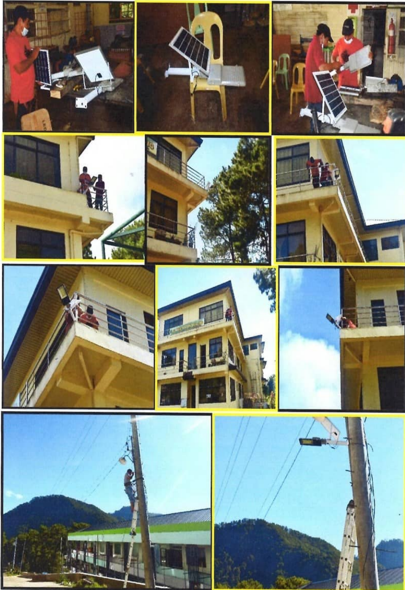
Assembly and installation of solar panels at Tadian Campus (March 2022)
